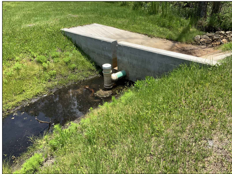
1602: • OUTFALL STRUCTURE IN GOOD CONDITION. MINOR DEBRIS BUILDUP.
