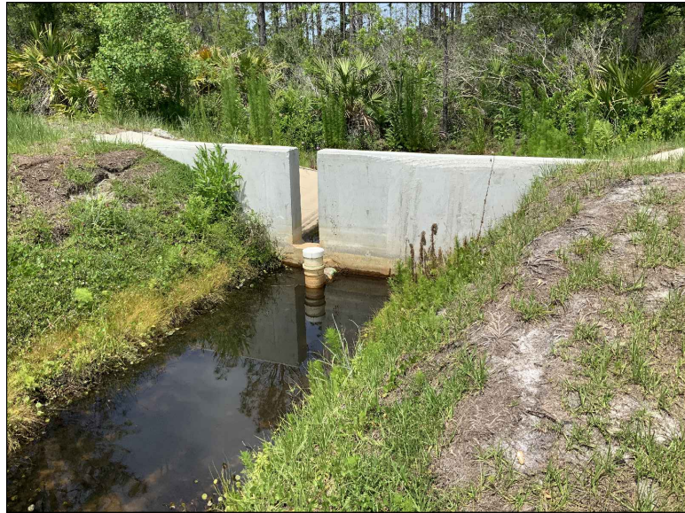
1902: • NORMAL WATER ELEVATION IS STAGING BEYOND ORIFICE OUTFALL.
