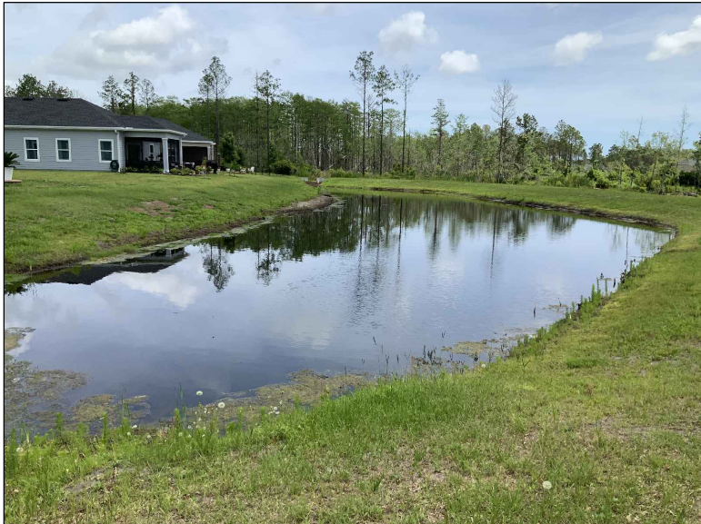
901: OVERALL POND BANKS HAVE MODERATE EROSION.
