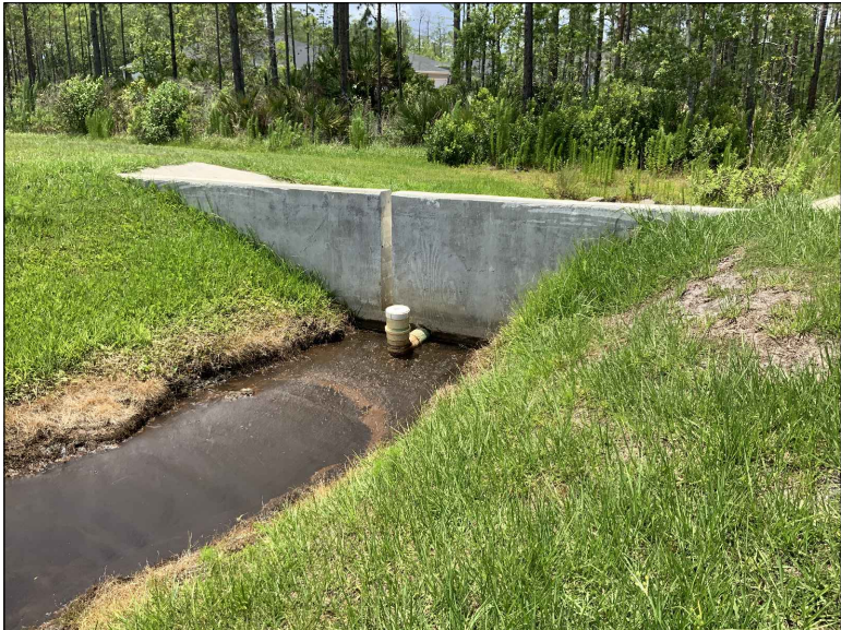
1803: • NORMAL WATER ELEVATION IS STAGING BEYOND ORIFICE OUTFALL.
