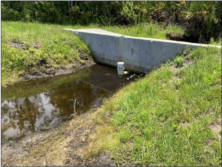
1702: • NORMAL WATER ELEVATION IS STAGING BEYOND ORIFICE OUTFALL.
