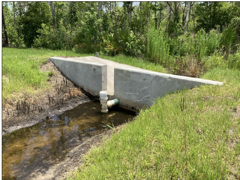
1301: • OUTFALL CONTROL STRUCTURE IN GOOD CONDITION AND AS PERMITTED.
