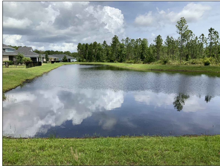
1002: • OVERALL POND BANKS IN GOOD CONDITION.
