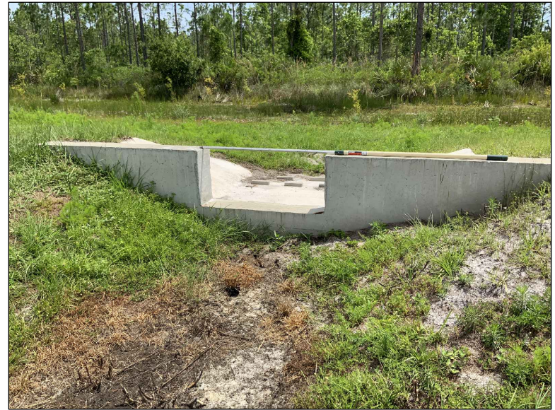
1003: • OUTFALL CONTROL STRUCTURE IN GOOD CONDITION.
