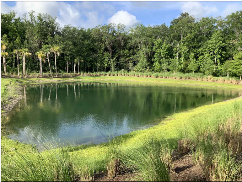
202: OVERALL POND AND VEGETATION LOOK TO BE AS DESIGNED AND IN GOOD CONDITION.
