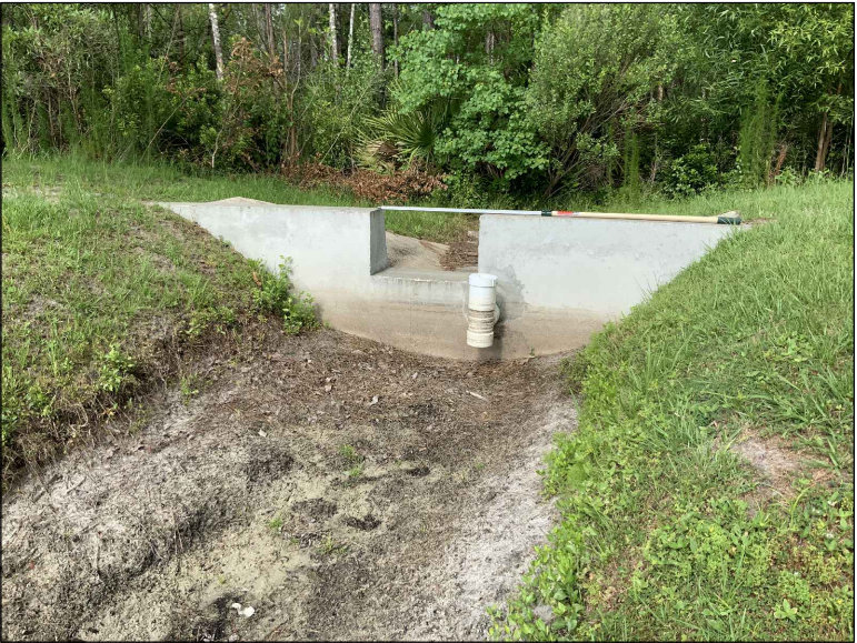
5-3: • OUTFALL CONTROL STRUCTURE IN GOOD CONDITION.
