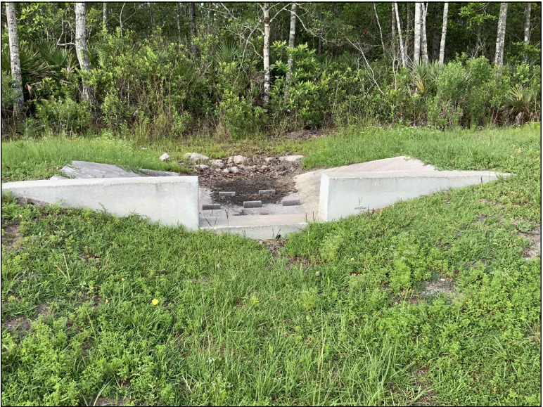
402: • OUTFALL CONTROL STRUCTURE IN GOOD CONDITION.
