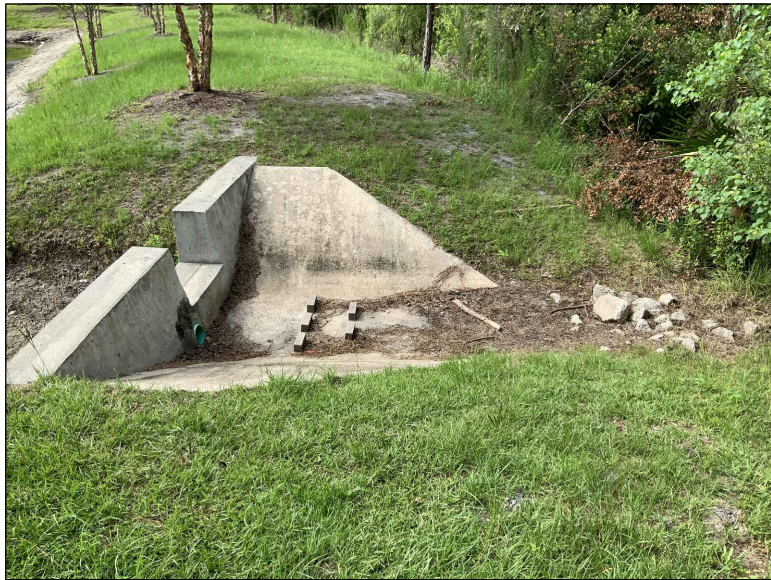
5-4: • OUTFALL CONTROL STRUCTURE HAS VERY MINOR DEBRIS BUILDUP.
