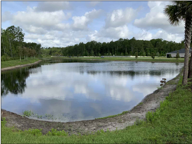
401: • OVERALL POND BANKS IN GOOD CONDITION.
