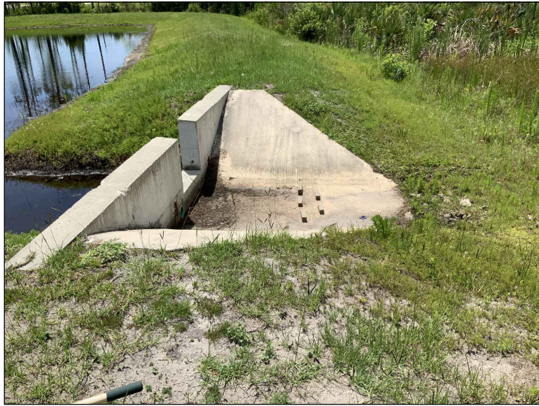
1101: • OUTFALL LOCATION IS FREE OF DEBRIS.
