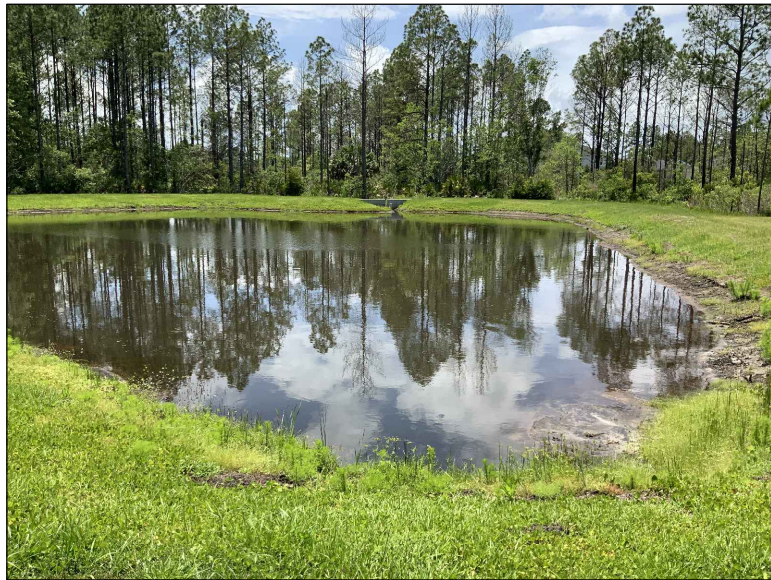
1601: • OVERALL POND BANKS IN GOOD CONDITION.
