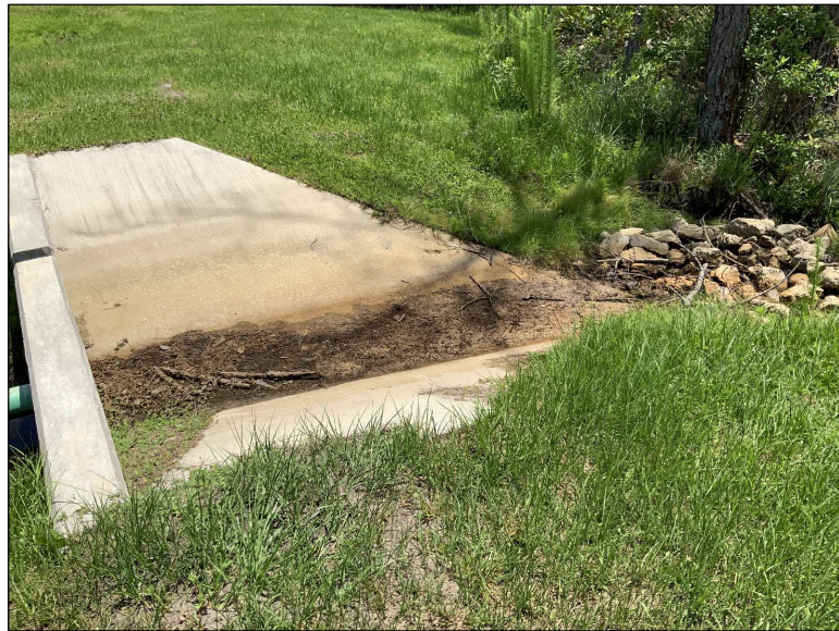
1603: • OUTFALL STRUCTURE IN GOOD CONDITION. MINOR DEBRIS BUILDUP.
