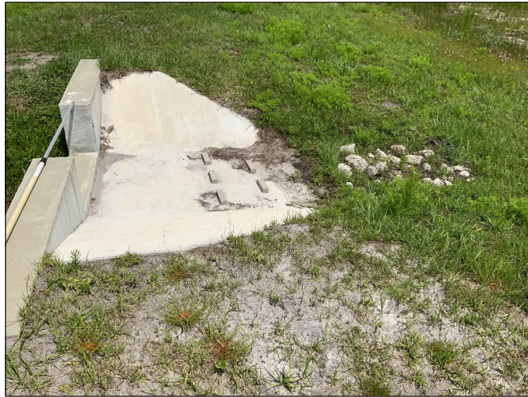
1001: • OUTFALL LOCATION FREE OF DEBRIS.
