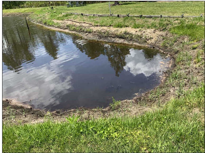
1503: • EXTENTS OF EXCESSIVE SLOPE AT END OF POND.
