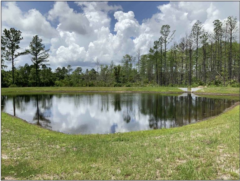
1102: • OVERALL POND BANKS IN GOOD CONDITION.
