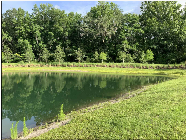
201: OVERALL POND AND BANKS IN GREAT CONDITION.
