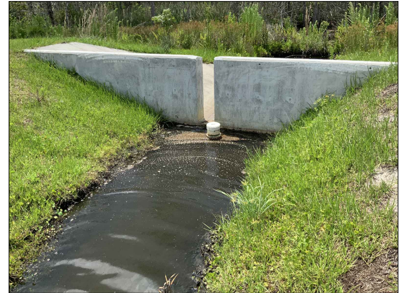
19-3: • NORMAL WATER ELEVATION IS STAGING BEYOND ORIFICE OUTFALL.
