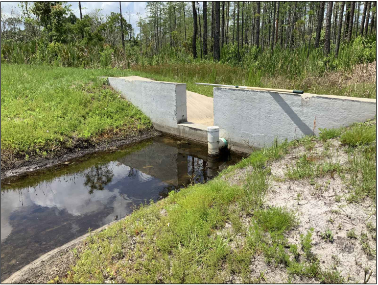
1103: • OUTFALL CONTROL STRUCTURE AS DESIGNED AND PERMITTED.
